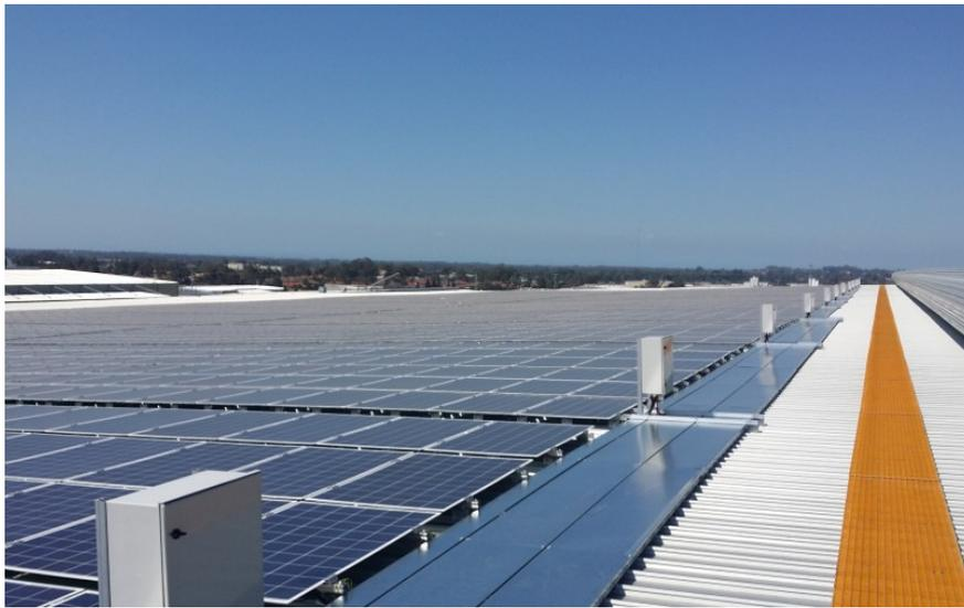
The Epho-built 1 MW solar system on Aldi Distribution Centre in Brendale, Queensland.
